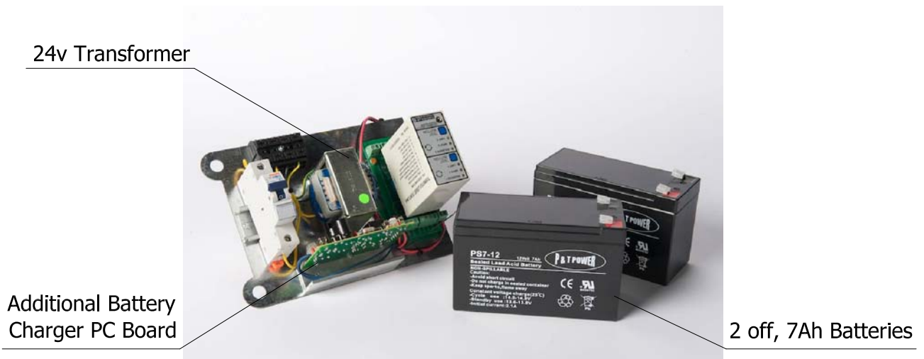
Figure 5.2: Turnstile Control Panel with Battery Backup Unit (with leads for batteries - not shown)
